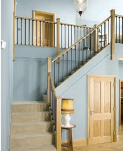
Metal balustrade with oak handrail
