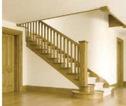
Cut and bracketed oak staircase
