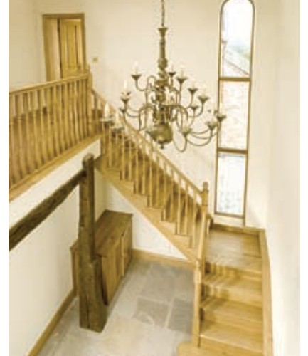
Cut and bracketed oak staircase
